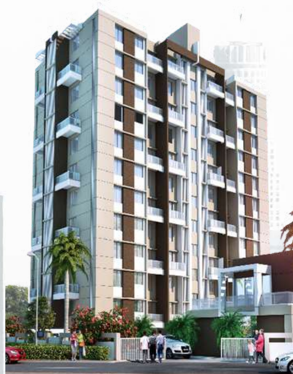
Harmony Homes (12 Floors)
