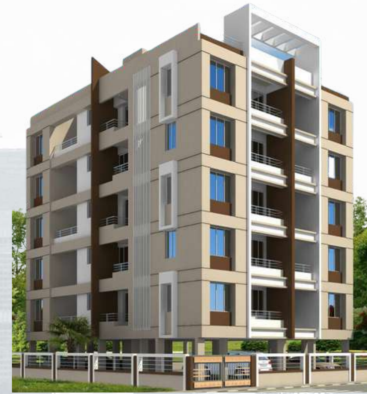
Alok Heritage (5 Floors)
